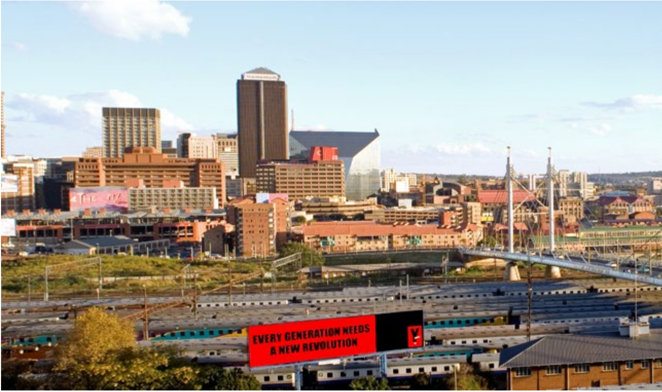
The Nelson Mandela Bridge crosses the Johannesburg Station shunting yards, linking the business districts of Braamfontein and Newtown.
